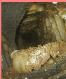
Figure 1.6 Cooling tower pack boroscope pictures
