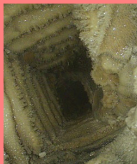
Figure 1.6 Cooling tower pack boroscope pictures
