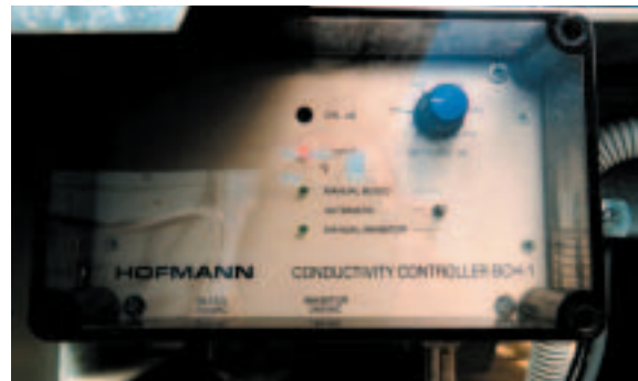
Conductivity meter: This meter measures conductivity of the water and controls a bleed-off valve to ensure the solids in the water do not exceed a pre-determined level
