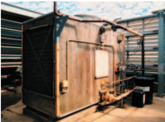
Wooden tower: An aged tower constructed largely of wood
