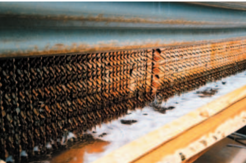
Cooling tower with basin exposed to sunlight: This cooling tower does not have sunlight protection to the side and basin of the tower
